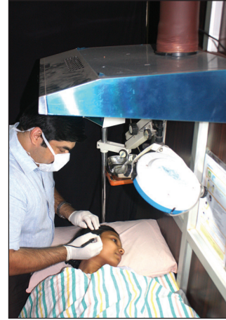
Figure 1: Commercially available kitchen chimney fitted right above the operation table about half a meter away from the patient
